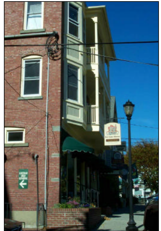
Apartment over stores, Katonah.
