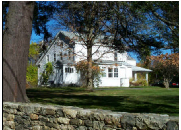
Single-family detached house on Haines Road, with intact stone wall and mature landscaping.
